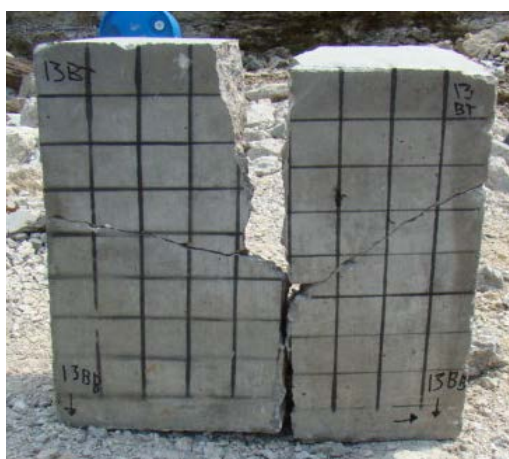
Figure 4.18: Block 13, back face after impact
